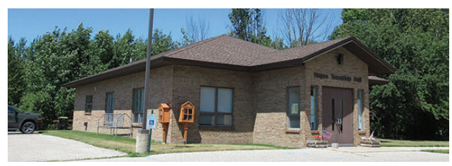
Hayes Township Hall, Charlevoix County
